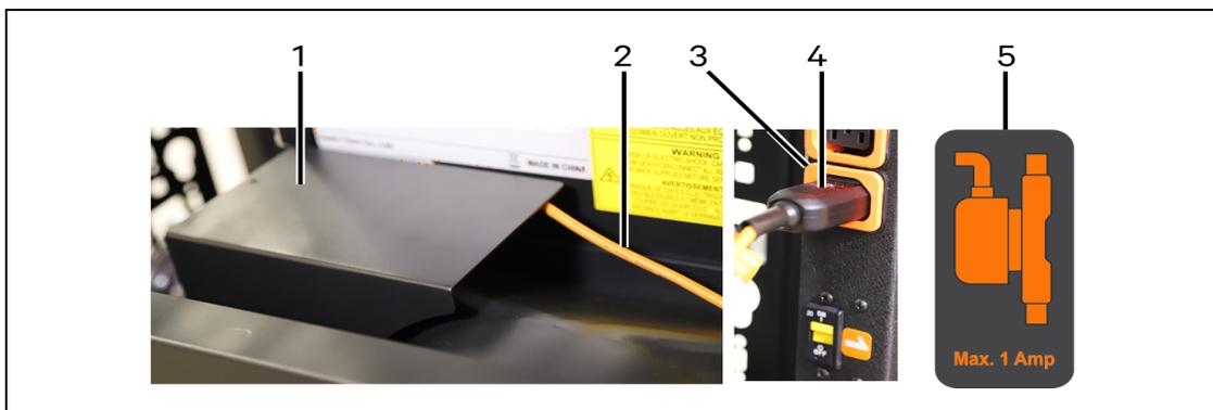
**Table 4.2 Condensate Pump Power Cord Routing, Connection Descriptions**
